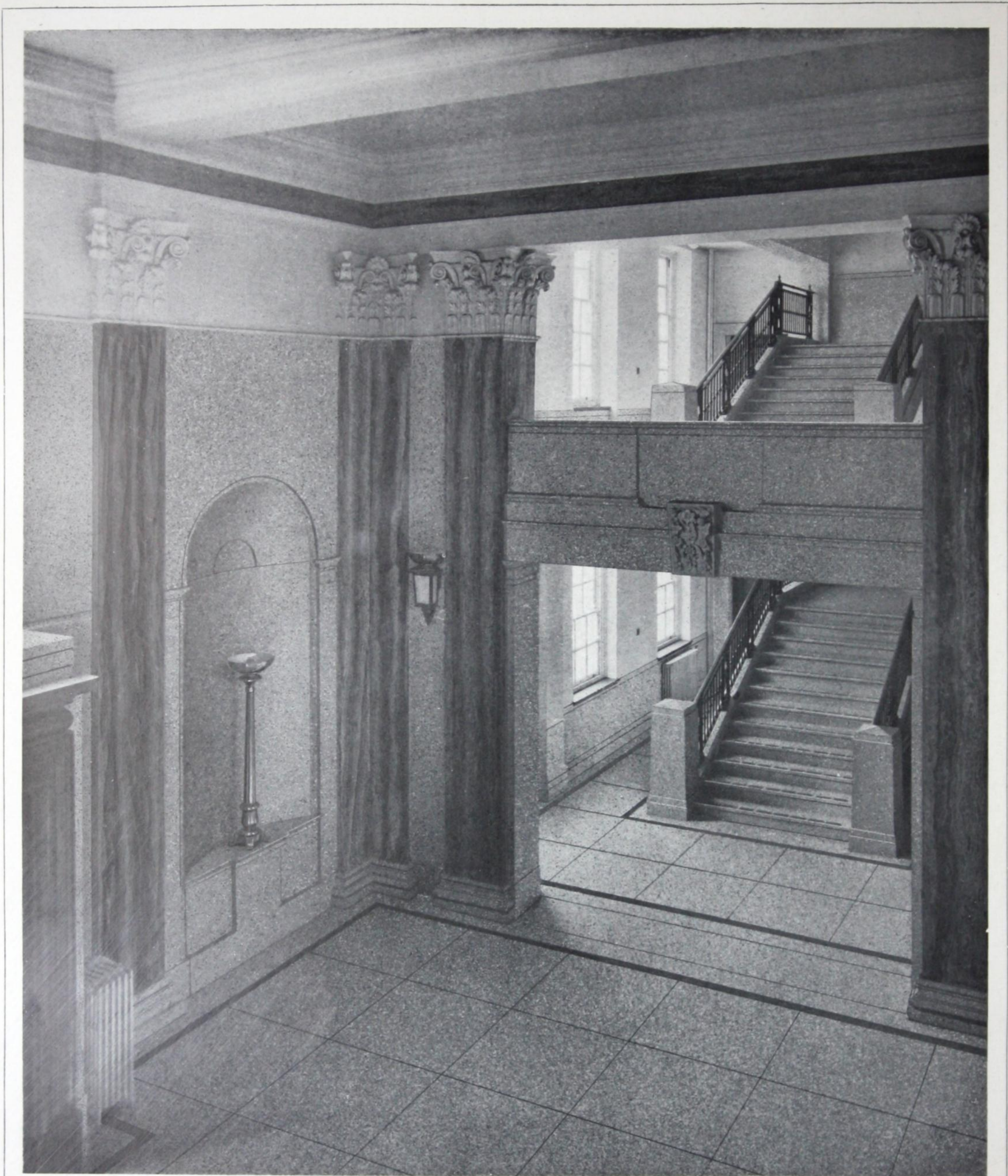
TERRAZZO COVERING TO WALLS, PILASTERS, NICHE, STEPS, PYLONS, BEAM, BASES AND CAPS, AND DADOES TERRAZZO SECTIONISED PAVING
