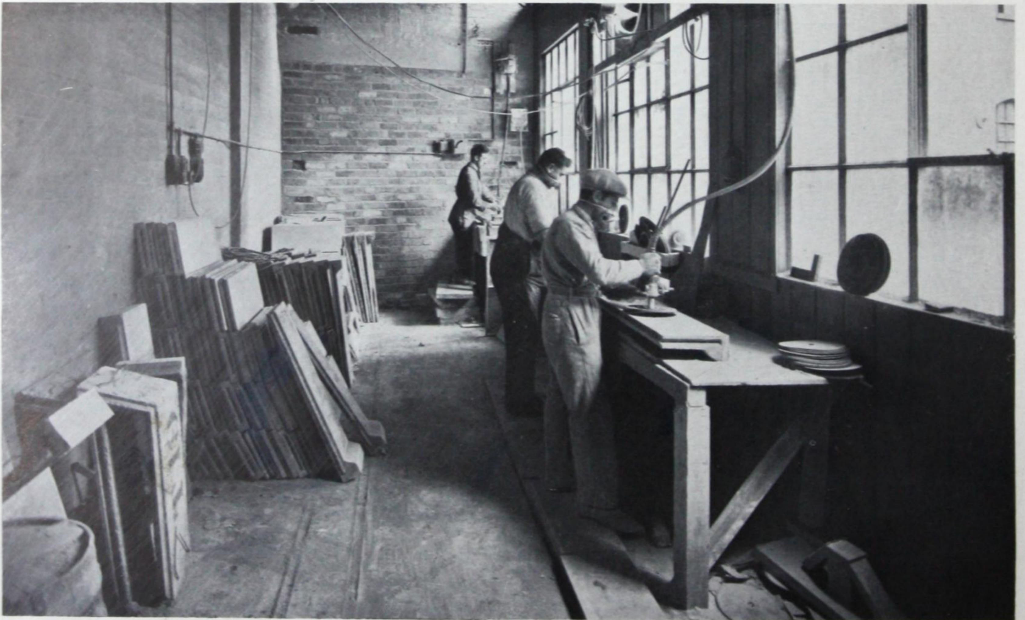
BIRMINGHAM WORKS, POLISHING SHED
