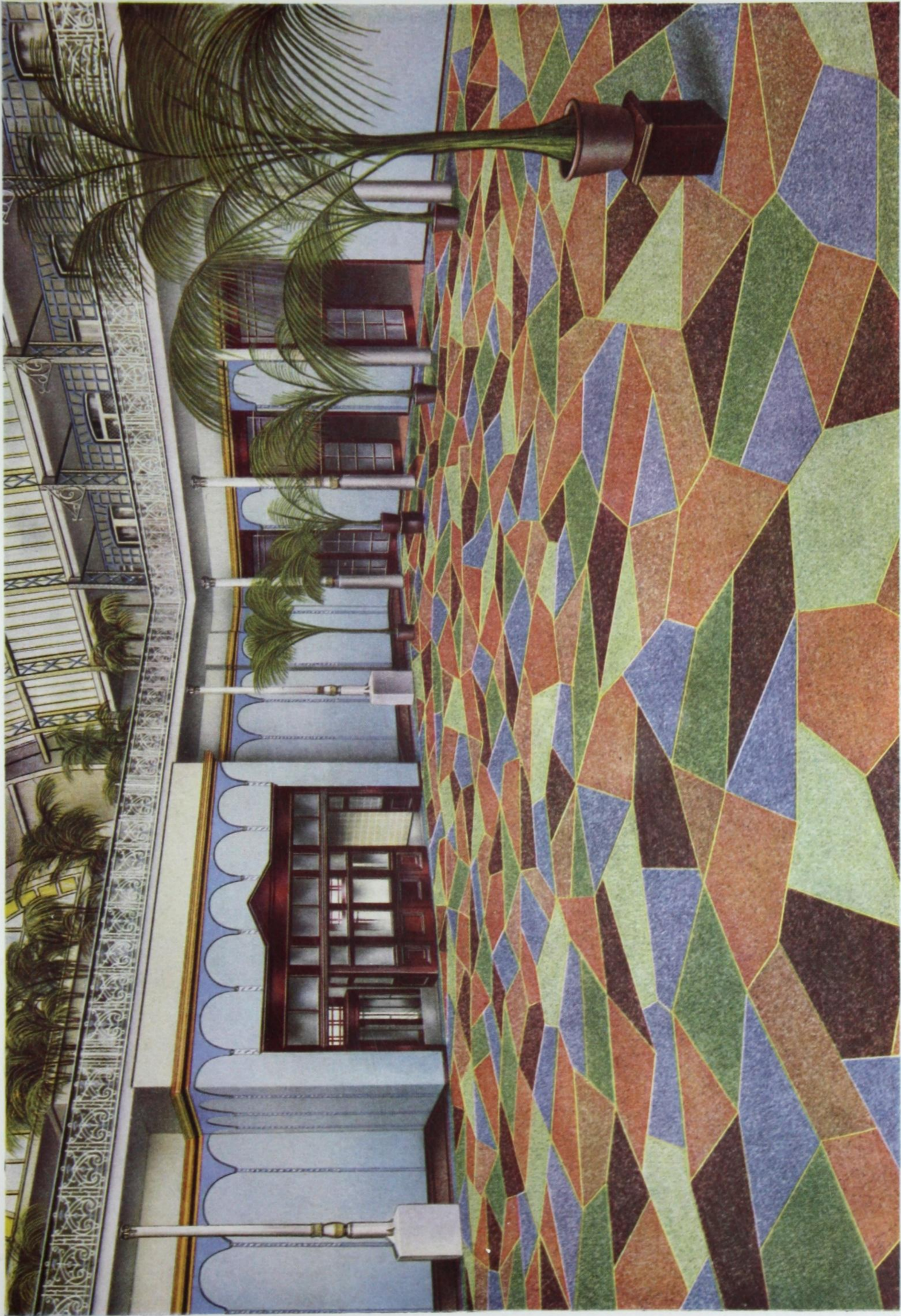
SECTIONISED TERRAZZO PAVING WITH BRASS DIVIDERS WINTER GARDEN, BLACKPOOL
