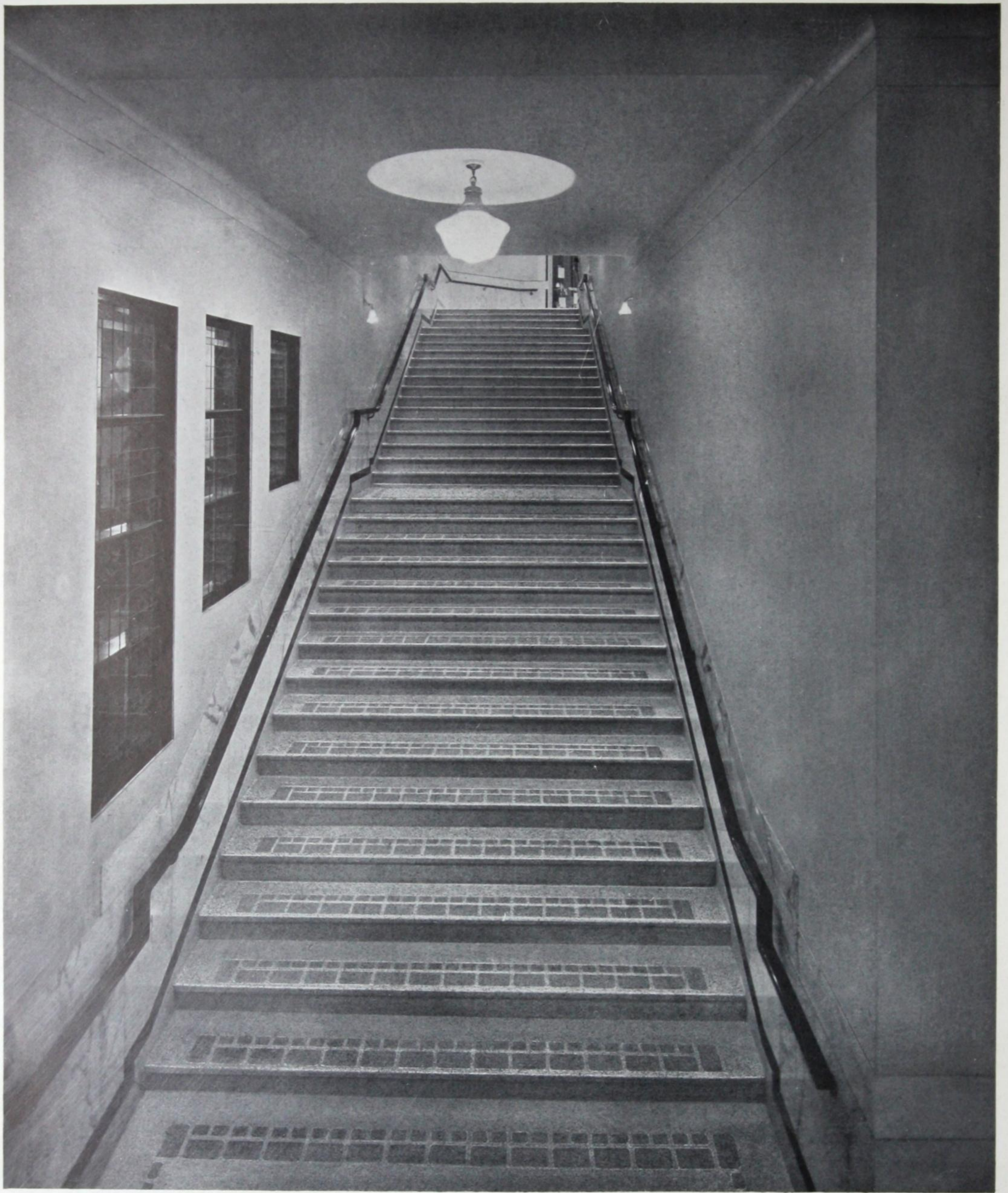
TERRAZZO STAIRCASE WITH TERRAZZO ALUNDUM NON-SLIP INSETS SELFRIDGES, LONDON
