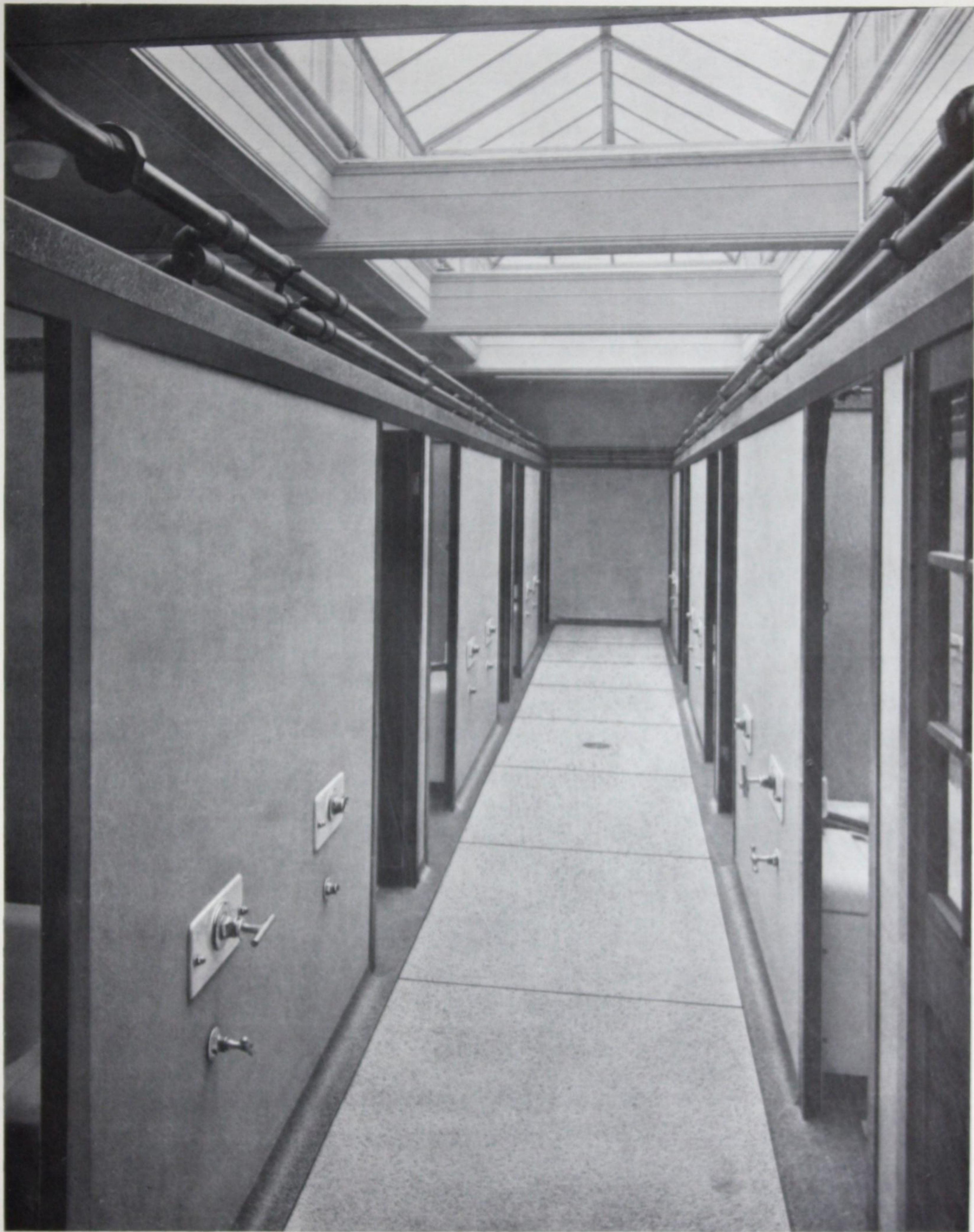
SECTIONISED TERRAZZO PAVING PRECAST TERRAZZO PARTITIONS DIESPEKER'S PATENT SYSTEM OF BRONZE METAL DOORPOSTS NEWCASTLE-ON-TYNE SLIPPER BATHS
