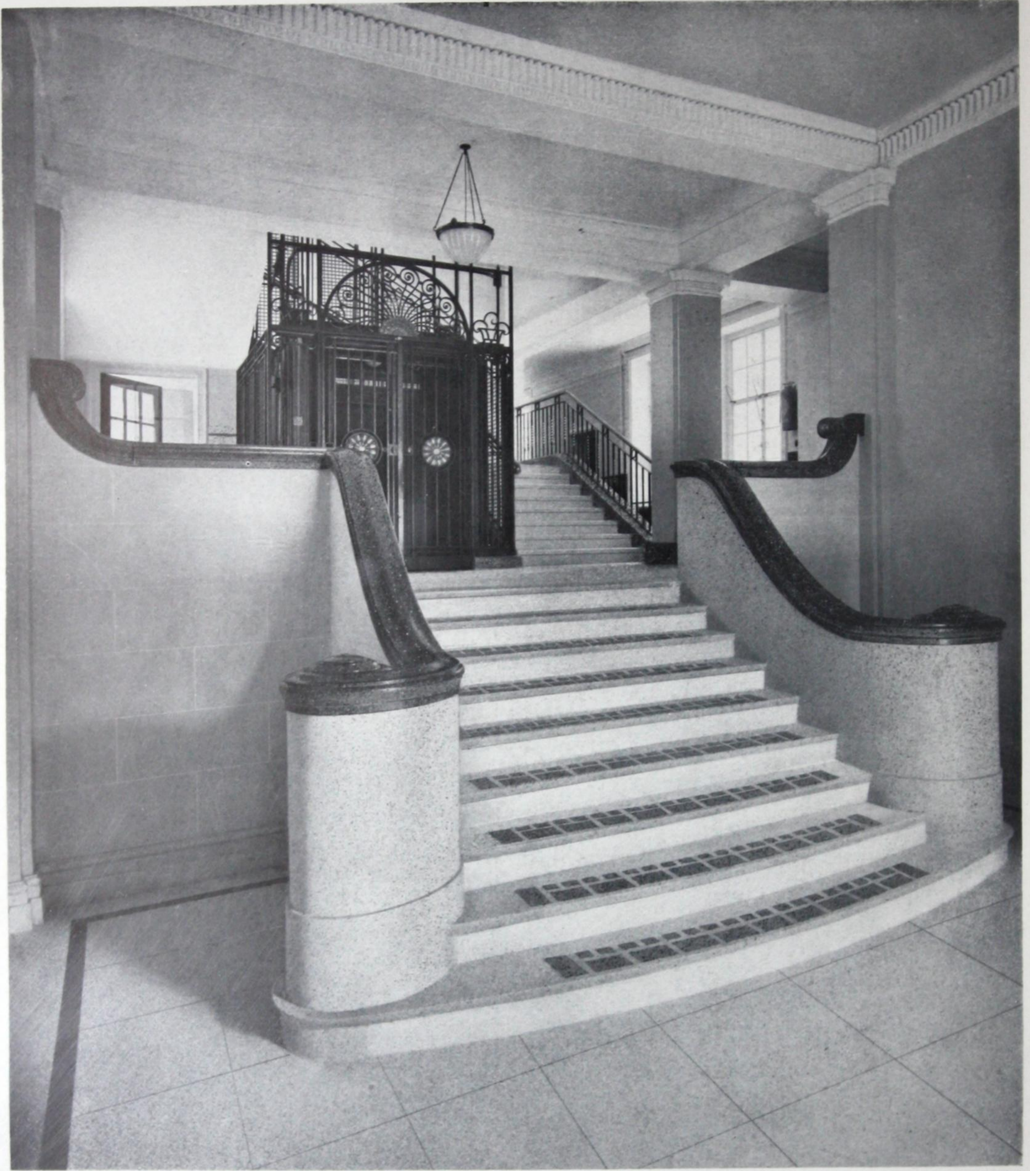
TERRAZZO STEPS, NEWEL WALL, MOULDED BALUSTRADE, NEWEL CAPS & MOULDED HALF CAPS, TERRAZZO TILE PAVING
